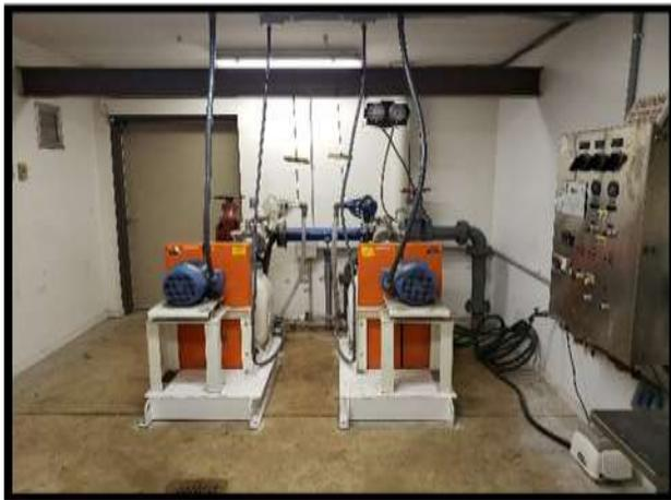
At the time of construction, the average flow was projected to be 17 gpm. With the addition of the Sunnyside and Ashley Heights Subdivisions, the current flow to the lift station averages 40 gpm. With this added flow, the station began to operate near maximum capacity. Given the capacity issues, age, and a lack of available repair parts, staff initiated a plan to remove the existing pumping equipment and upgrade utilizing pumping equipment removed from Lift Station #19 and
